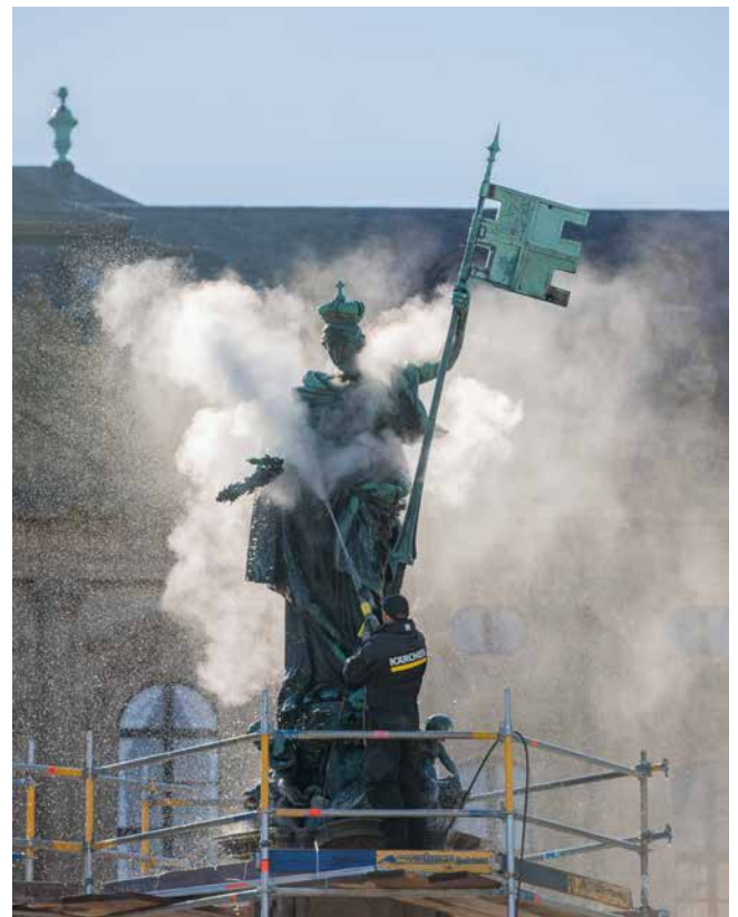
It's not made from stone, but from bronze. Having removed the millimeter-thick layer of limescale, the Franconia fountain shows its true face once again.
